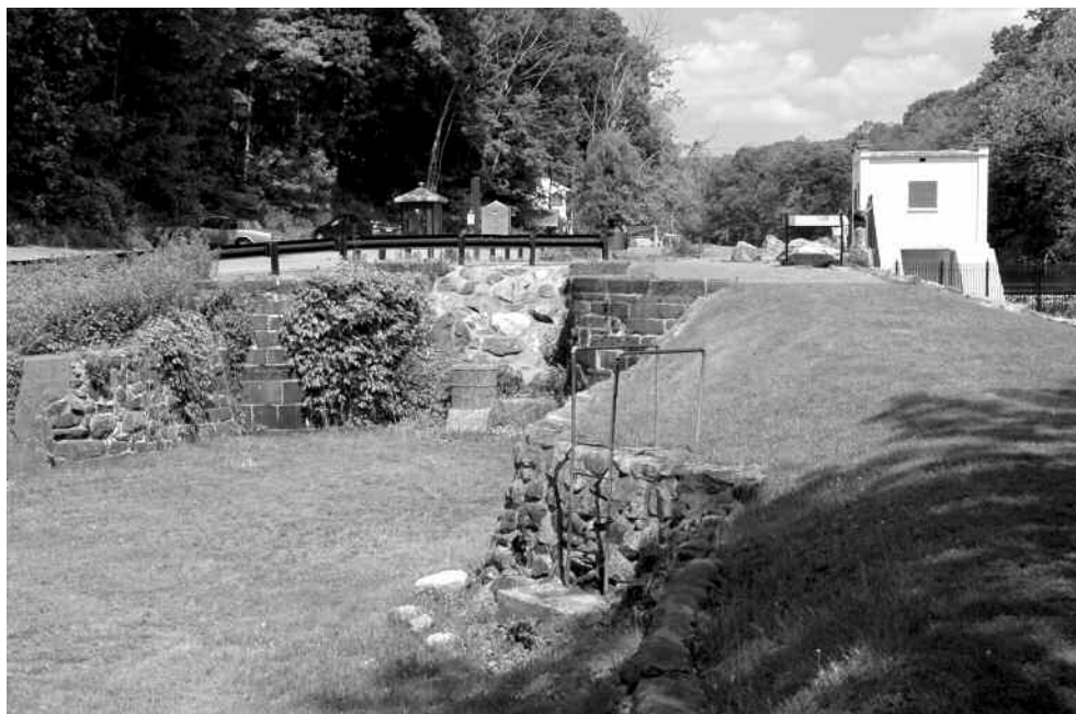
The lock at Saxton Falls is one of the most visibly intact locks on the overall Morris Canal.
