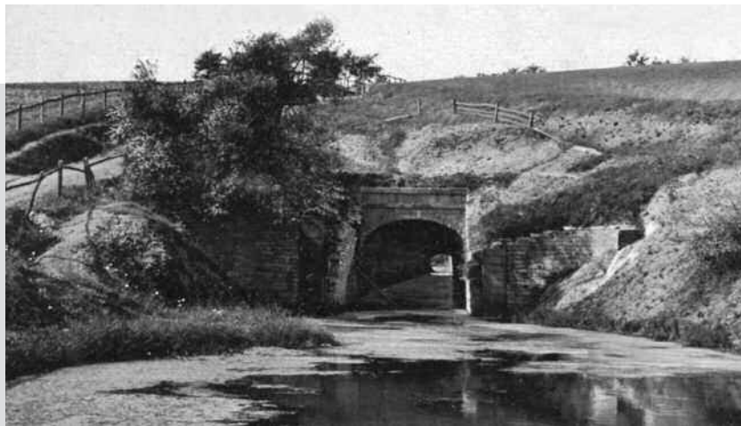
Historic view of Union Canal tunnel.
