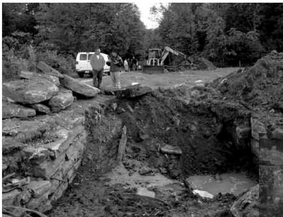
At Wharton a test trench dug across Lock 2 East revealed that below grade the lock walls are substantially intact. (Left) In the turbine chamber at Plane 2 East in Ledgewood, archeologists examined the tailrace arch to design masonry repairs. (Below).
