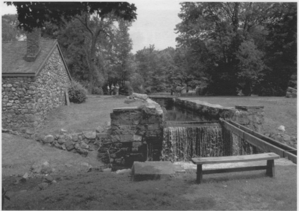
Waterloo's picturesque Morris Canal lock was a combination lock and aqueduct and spanned the nearby gristmill's tailrace. The blacksmith shop is to the left of the lock.
