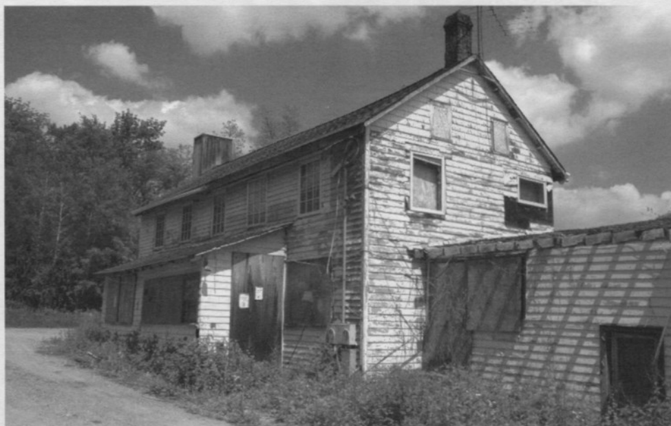
Present-day view of the deteriorated locktender's house at Lock 4 West.
