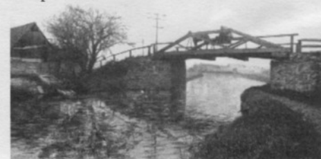
Baker's Bridge, Morris Canal, Kenvil, NJ
