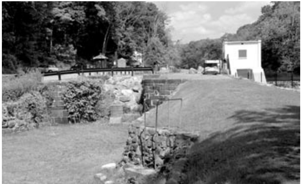
Present-day view of Lock 5 West (center) within the Saxton Falls section of Stephens State Park.
