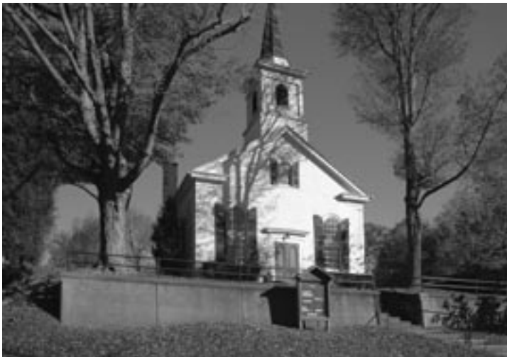
The well-preserved Waterloo United Methodist Church looks virtually as it did at the time of its 1859 construction.
