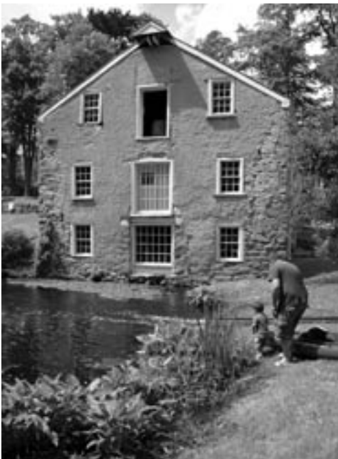
The old wooden hoist wheel remains in the loft of Smith's Store. When the canal was active merchandise could be unloaded from boats and lifted through the large doors on each level of the building.
