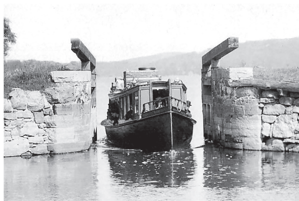
ABOVE: A steamer passes through the stop gate before entering the small basin that separated the lake from the Brooklyn Lock.
