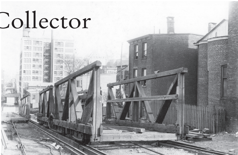
Two cradle cars stand idle on Inclined Plane 12 East in Newark. This was one of the canal's three double-tracked planes with counterbalanced plane cars, one going up while the other came down.
