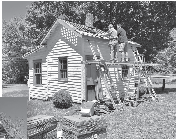
ABOVE: In October contractors worked to apply a new wood shake roof to the Kingston Toll Collector's House.
