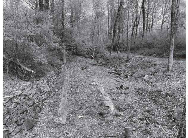
The landscape here at Plane 7 West is so altered that this short section of stone sleepers at the very bottom of the plane is the only place we can see its original configuration.
