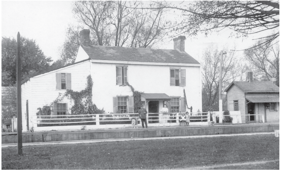
Today the lock and Lock Tender's House are part of D & R Canal State Park
