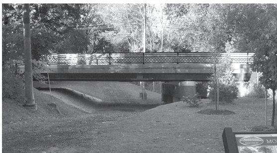
BELOW: The Berkeley Avenue Bridge, seen here from the east, was the first generation steel bridge built in 1906. It was replaced with a through plate girder bridge in 1922, and demolished in 2016.
