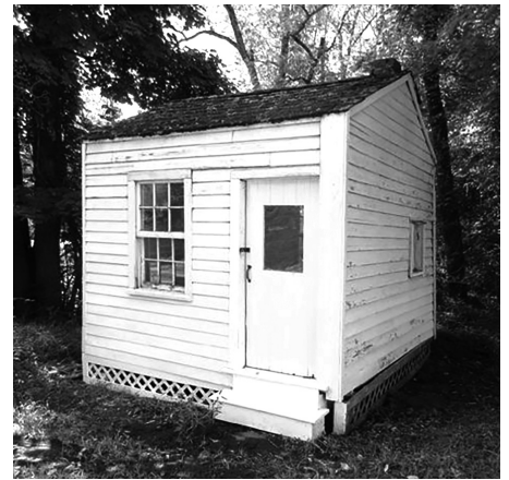
The Griggstown Bridgetender's Station shown here after repair work had been completed.
