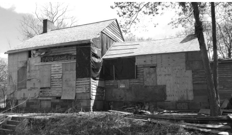
The Collins House in progress with new cedar shake shingle roof.
