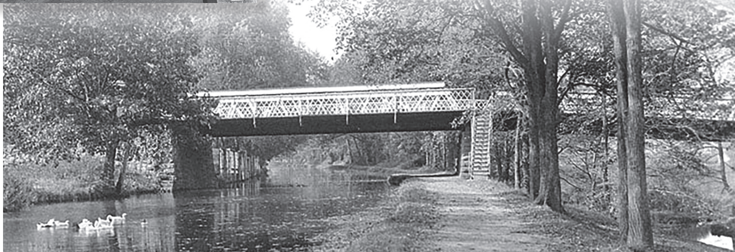
LEFT: To preserve this historic setting new Berkeley Avenue Bridge was built with cantilevered sidewalks, decorative railings and stone abutments and piers.
