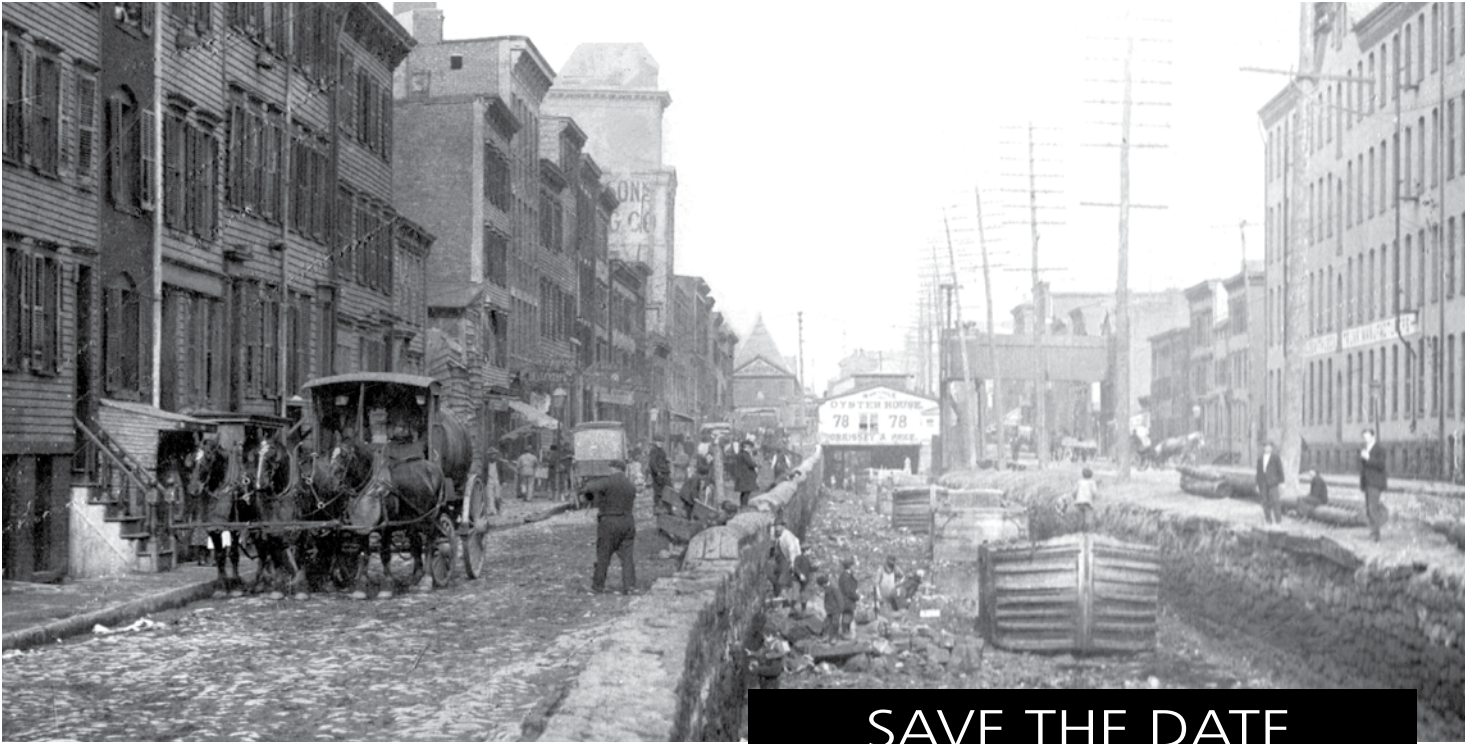
This enlarged view shows workers in the canal bed and activity along both sides of Canal Street in great detail. On the far right a bystander with a hand-held camera takes his turn at capturing the on-going repairs and cleanup.
