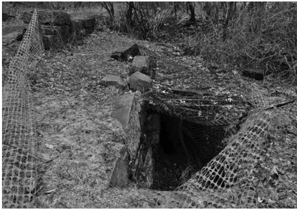
The top of the turbine chamber shaft before restoration.
