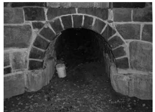
To solve the problem, masons added new concrete footings, realigned the arch and repointed all the stonework.
