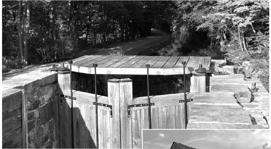
ABOVE: At the lower end of the lock, the platform has been built to hold the machinery that will be used to crank the miter gates open and closed. The four vertical iron rods seen in the picture are attached to the wicket gates that were opened to empty the lock.
