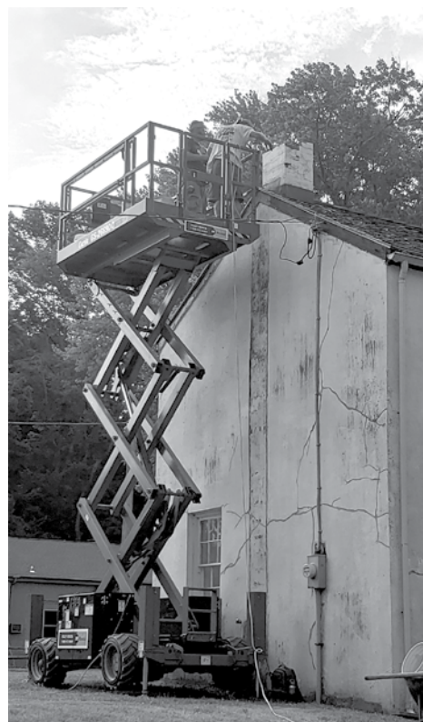
Workmen disassemble the old chimney,
