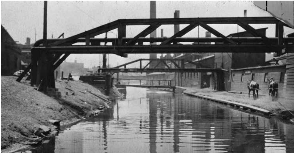
This historic photo shows the Balbach Smelton and Refining Company that once stood along the Passaic River in the Ironbound section of Newark. The Morris Canal passed through the center of the plant causing problems for both the canal and zinc company. In the picture above, utility lines are seen passing up and over the canal while the towpath is relegated to a narrow strip between the canal and the factory buildings, a situation that was bound to take lawyers to straighten out. This property is now part of Newark's Riverside Park.
