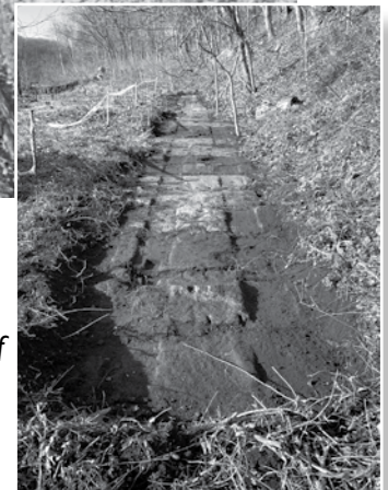
Newly uncovered sleeper stones.
