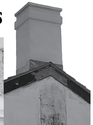
The completed chimney and flashing repair.
